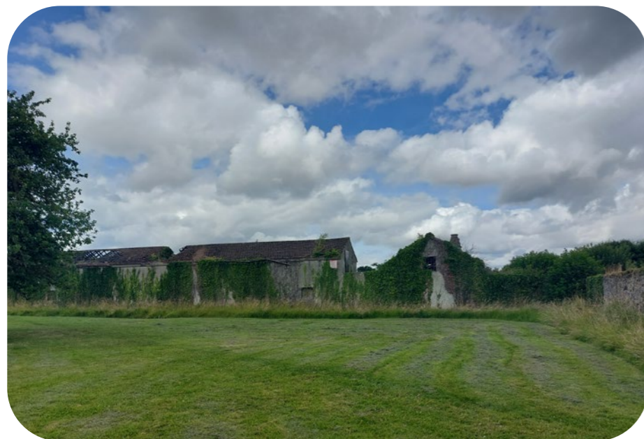
Figure 59; Existing Photo of current conditions
