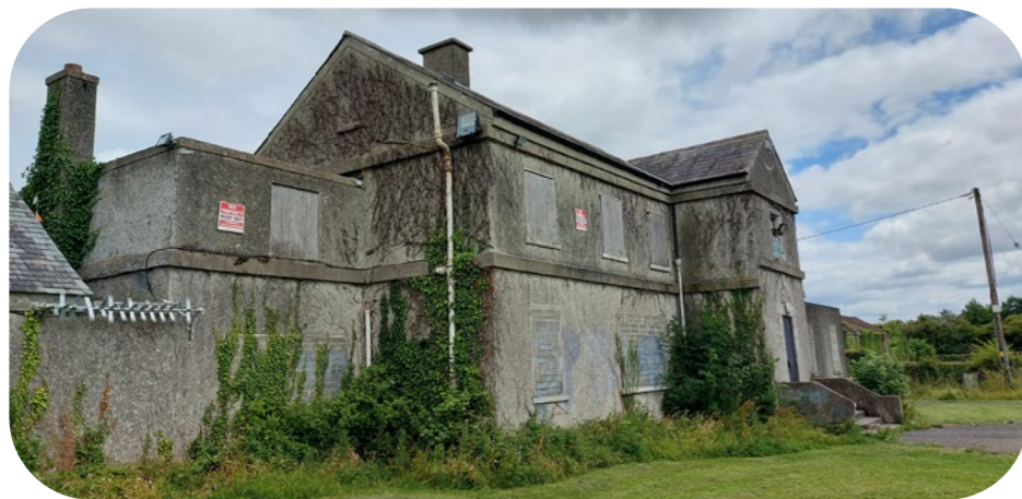
Figure 56; Existing Photo of current conditions
