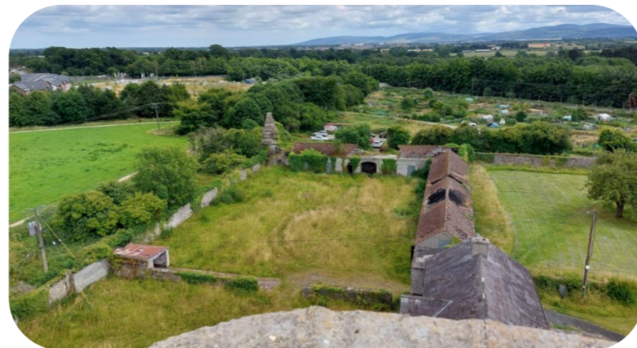
Figure 7; View from top of barn (looking east)
