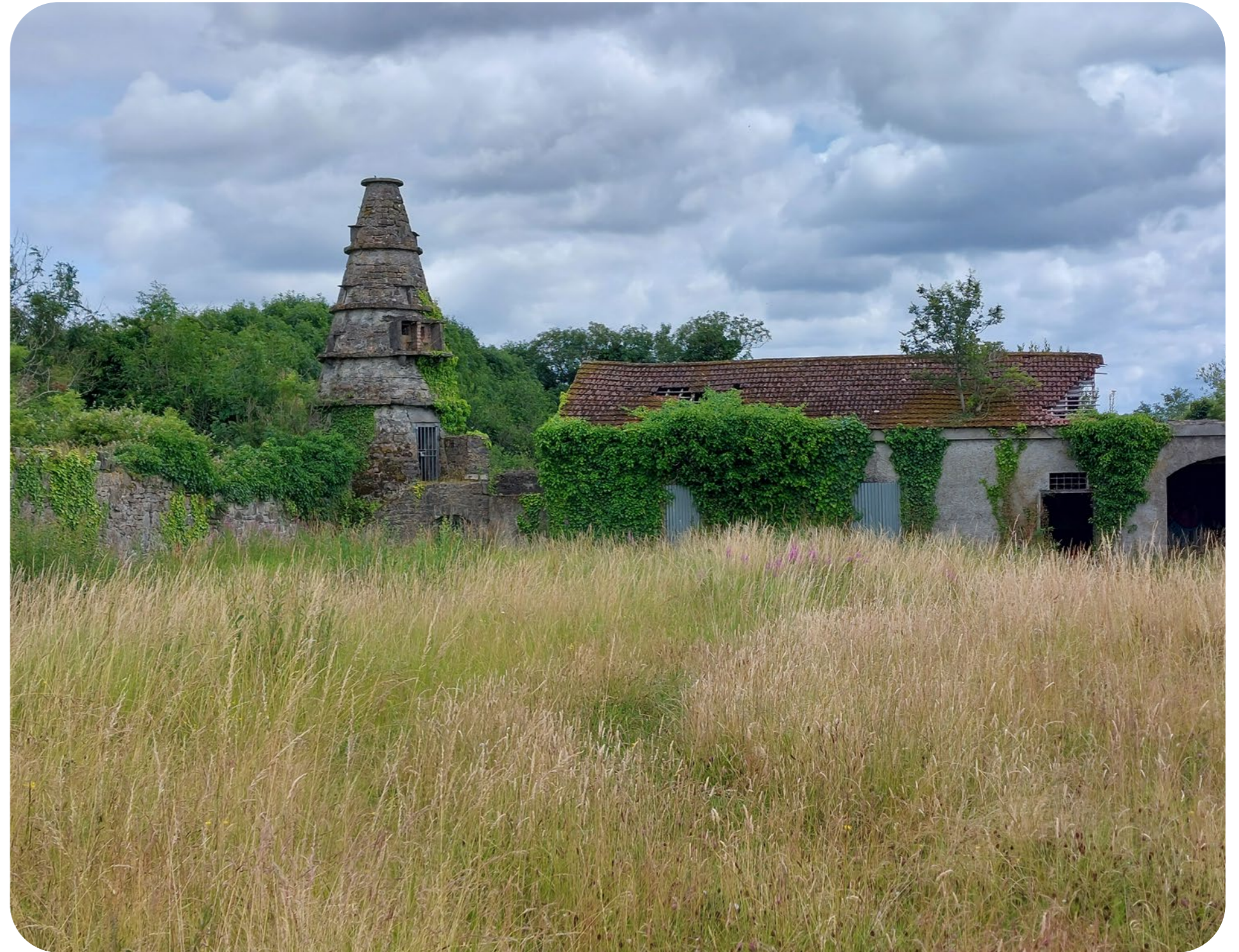
Figure 53; Existing Photo of the South Dovecote current condition
